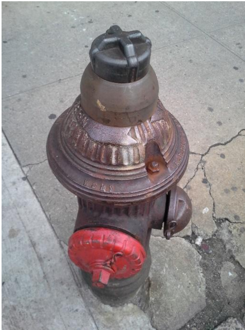
Figure 5: A fire hydrant with a “custodian”-style plus-shaped lock installed on top, New York City, NY. (Photo by author.)
