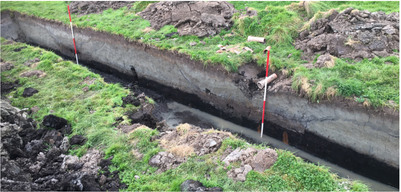
Fig. 14. Photo of the section of the embankment structure in the first excavation trench (source Bakker 2022b, Fig. 9). The ranging rods (2 m) are positioned in the middle of the ditches on either side of the ridge. The clay-and-peaty fill of these ditches has partly sunken into the peat subsoil.
