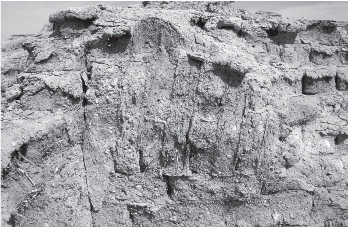
Fig. 7. Threshing remains are clearly visible in the mud bricks and mortar from a wall in Roman Karanis (Fayum, November 2003) (photo R.T.J. Cappers).
