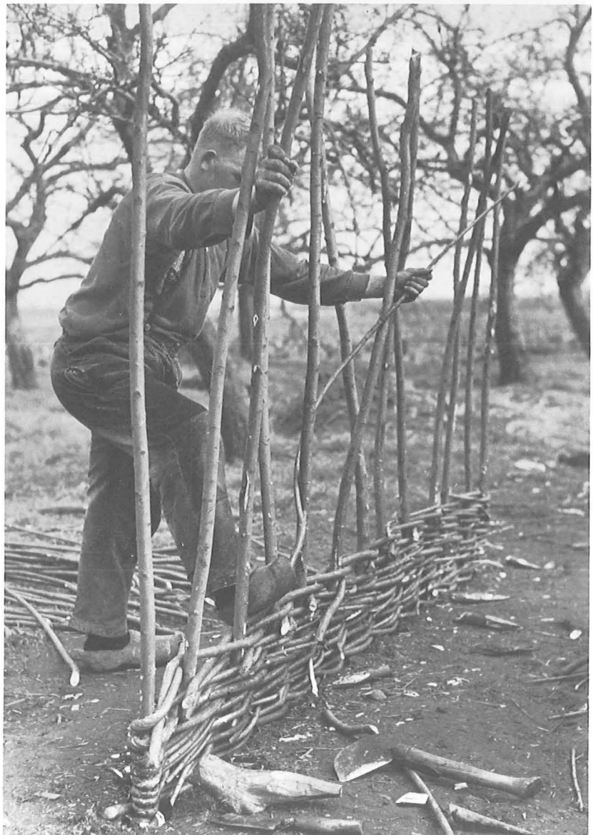
Fig. 38. A modern hurdle of Salix rods being made by A. van Weverwijk of Culemborg, near the River Lek in the riverine region of the Central Netherlands. Photo taken on April 14th, 1949 by Ir. W.D.J. Tuinzing. In the foreground the tool kit of the hurdle-maker: wood-cutting knife, a kind of wooden hammer and billhook.
