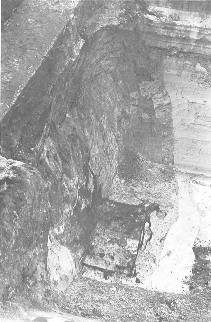
Fig. 11. Well I, with traces of the wooden sheet-piling.
