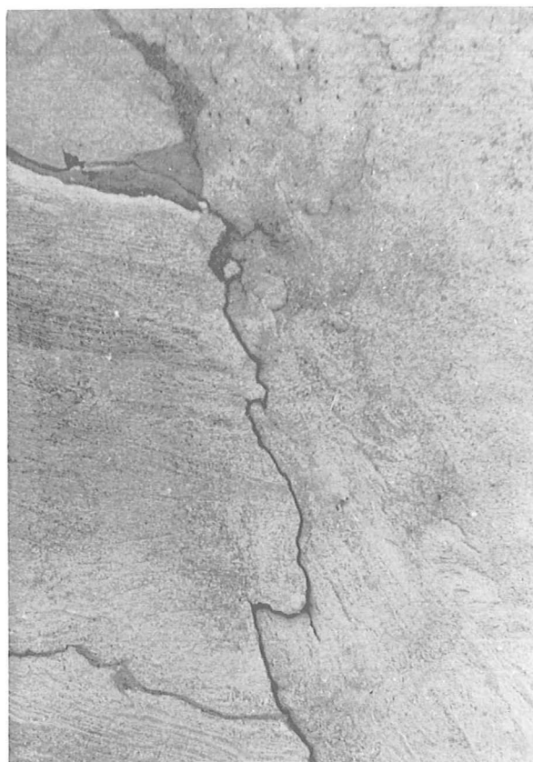
Fig. 14. Basin I, detail of the upper part of the wall, where locally undercutting had taken place (photo 1/3 of actual size).
